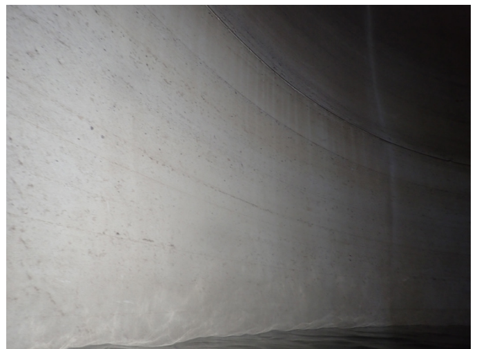
60 Interior Walls Having Good Adhesion Value Of The Protective Coating And A Mild To Moderate Stain/ Biofilm
