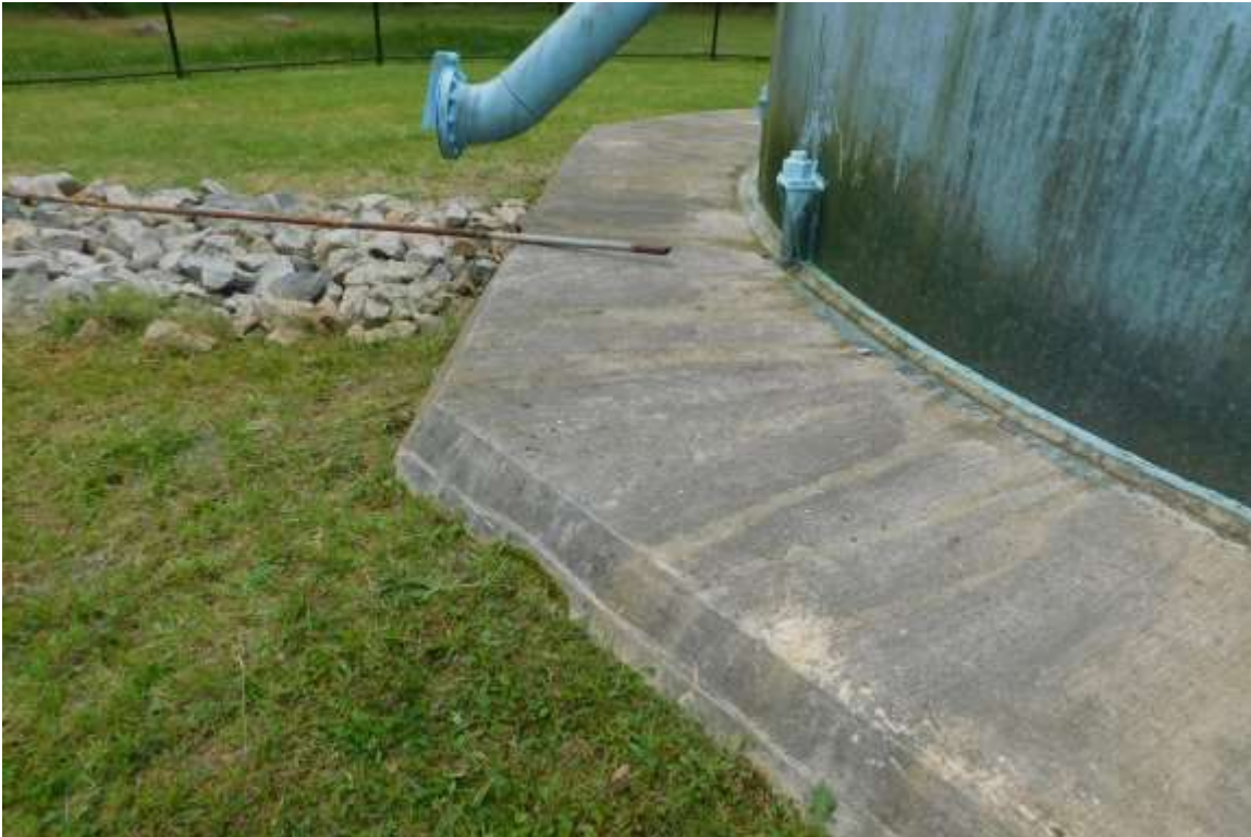
Photo shows the condition of the foundation. We recommend sealing the foundation with a sealant.
