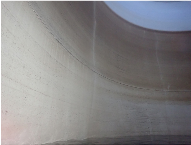
61 Interior Walls Having Good Adhesion Value Of The Protective Coating And A Mild To Moderate Stain/Biofilm
