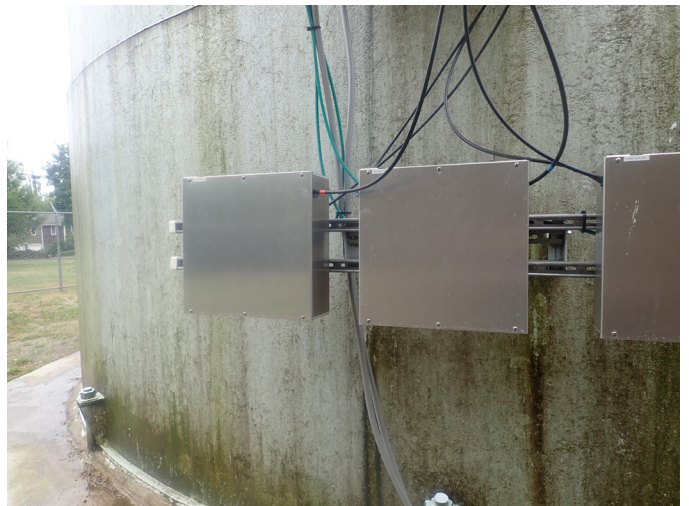
6 Securely Installed Cellular Communication Equipment
