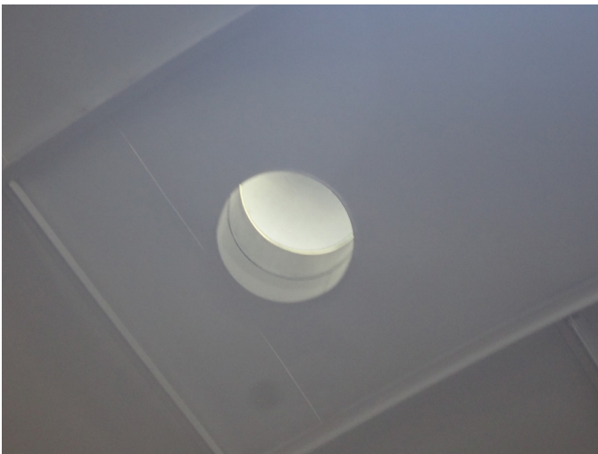
69 Unobstructed Vent Penetration
