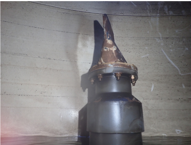
51 Unobstructed Rubber Influent Check Valve
