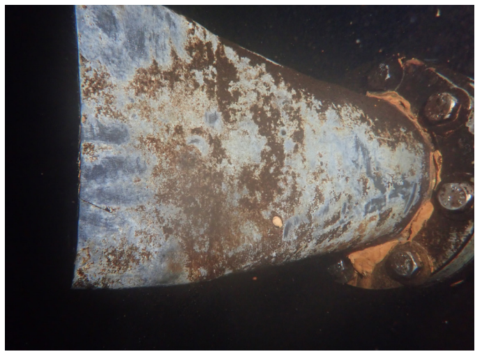
54 Mild Corrosion On The Metal Components Of The Water Circulation Pipe
