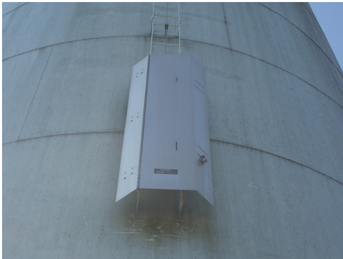
15 Ladder Guard Secured With A Lock
