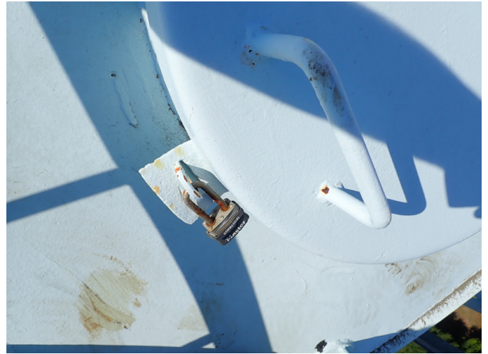
32 24" Inside Diameter Hatch Closed And Secured With A Lock
