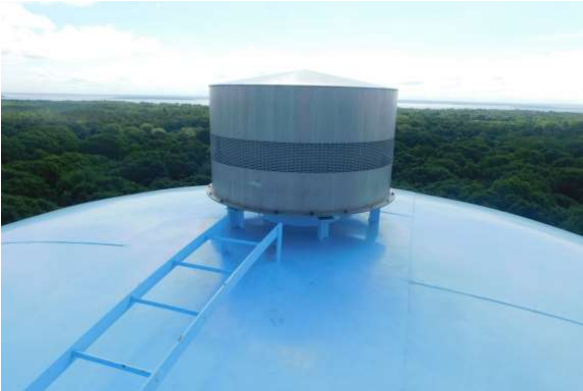
Photo shows the existing roof vent, which appears to be in good condition.
