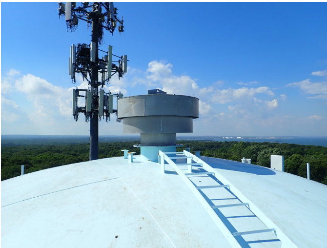
27 Vent Access Ladder Having Good Adhesion Value Of The Protective Coating
