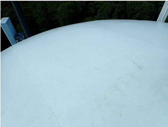
19 Roof Having Good Adhesion Value Of The Protective Coating And A Non-Uniform Accumulation Of Mildew
