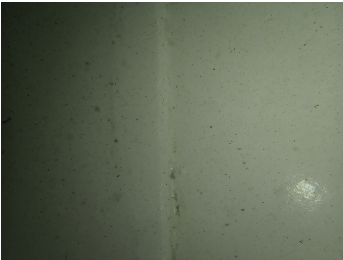
39 Floor Having Good Adhesion Value Of The Protective Coating And A Mild Stain/Biofilm
