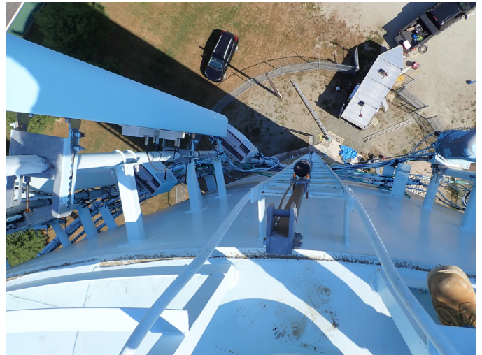
14 Ladder And Fall Prevention Device
