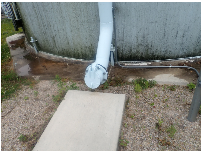
17 Overflow Pipe Terminating Above A Concrete Splash-Pad And Having A Secure Flap-Valve
