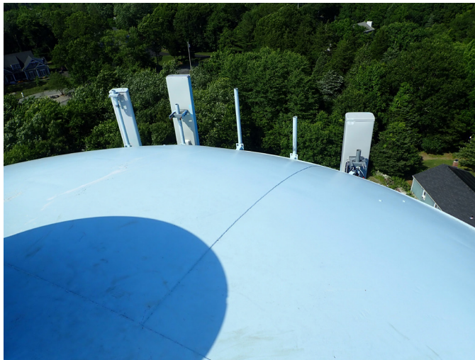
21 Roof Having Good Adhesion Value Of The Protective Coating And A Non-Uniform Accumulation Of Mildew
