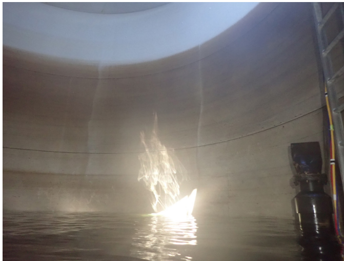
63 Interior Walls Having Good Adhesion Value Of The Protective Coating And A Mild To Moderate Stain/Biofilm
