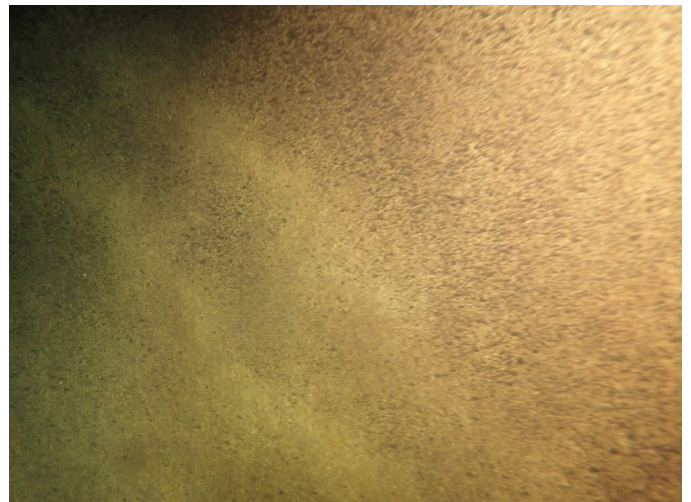
58 Interior Walls Having Good Adhesion Value Of The Protective Coating And A Mild To Moderate Stain/ Biofilm
