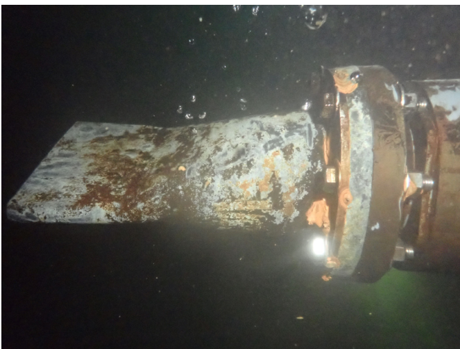
53 Mild Corrosion On The Metal Components Of The Water Circulation Pipe
