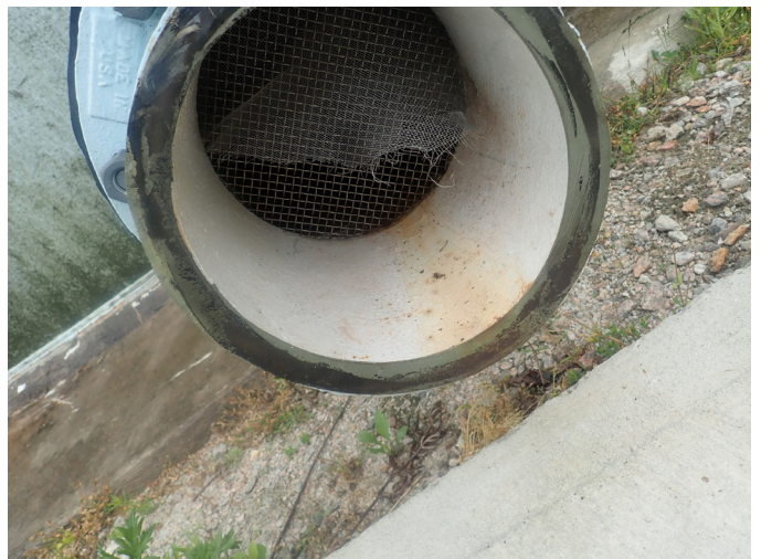
18 Torn/Dislodged 16-Mesh Overflow Screen
