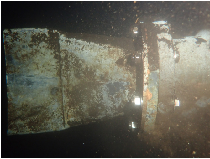
49 Unobstructed Rubber Influent Check Valve
