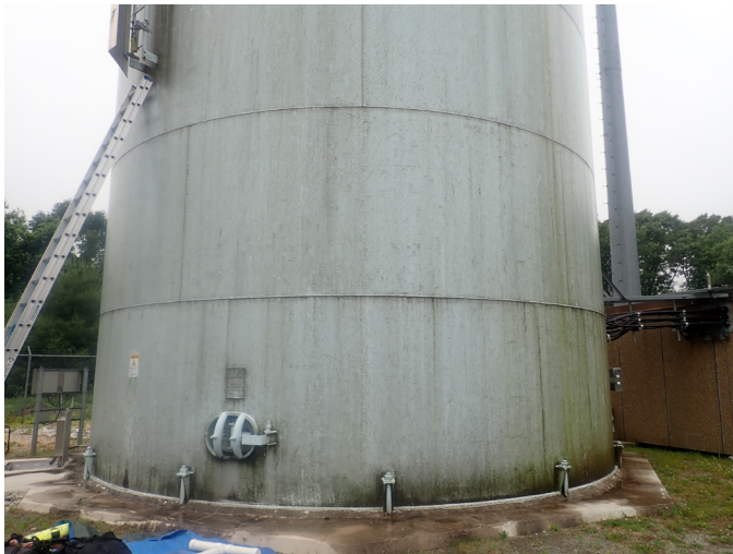
3 Exterior Walls Having Good Adhesion Value Of The Protective Coating And A Non-Uniform Accumulation Of Mildew
