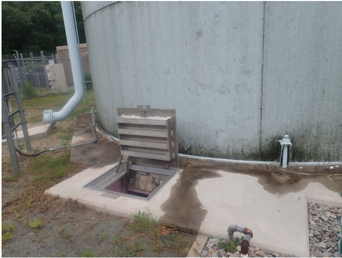
1 Exterior Walls Having Good Adhesion Value Of The Protective Coating And A Non-Uniform Accumulation Of Mildew
