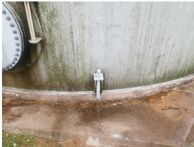
9 Exposed Foundation Having Tight Cracks And Anchor Bolt Assembly Having Good Adhesion Value Of The Protective Coating
