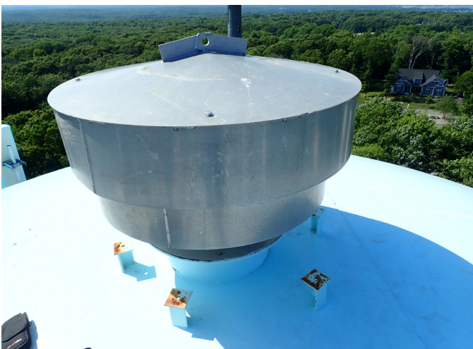
23 Pedestals Around The Vent Having Surface Corrosion
