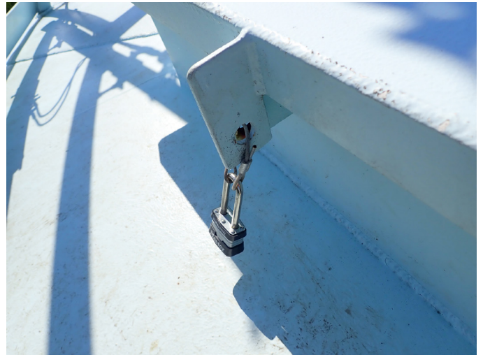
34 36" By 36" Hatch Closed And Secured With A Lock
