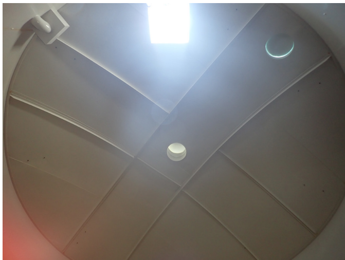
65 Overhead Having Good Adhesion Value Of The Protective Coating
