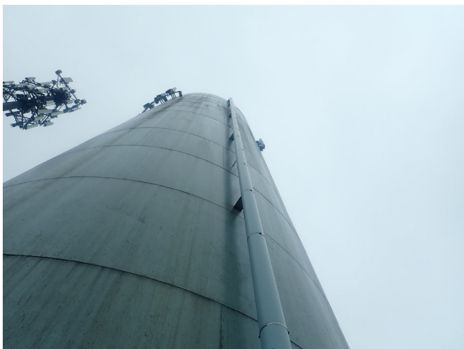
5 Exterior Walls Having Good Adhesion Value Of The Protective Coating And A Non-Uniform Accumulation Of Mildew
