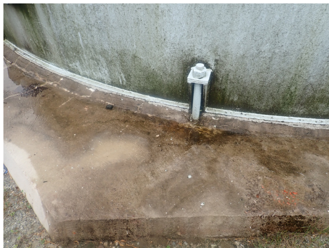
11 Exposed Foundation Having Tight Cracks And Anchor Bolt Assembly Having Good Adhesion Value Of The Protective Coating
