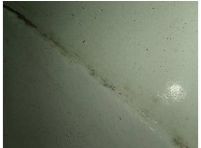
38 Floor Having Good Adhesion Value Of The Protective Coating And A Mild Stain/Biofilm
