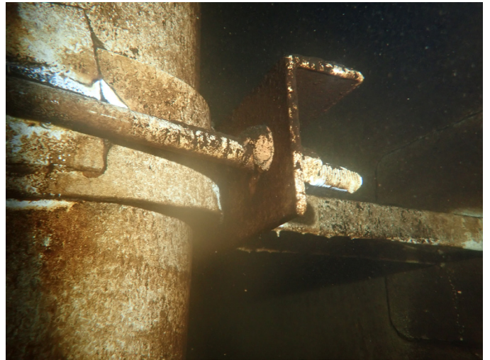
52 Mild Corrosion On The Metal Components Of The Water Circulation Pipe
