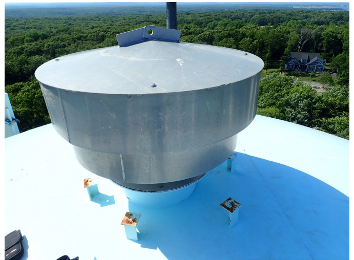
28 Secure Vent Assembly
