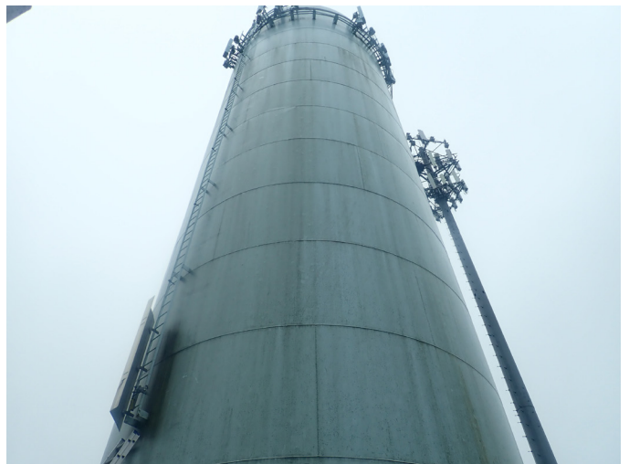
4 Exterior Walls Having Good Adhesion Value Of The Protective Coating And A Non-Uniform Accumulation Of Mildew
