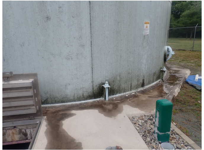
2 Exterior Walls Having Good Adhesion Value Of The Protective Coating And A Non-Uniform Accumulation Of Mildew
