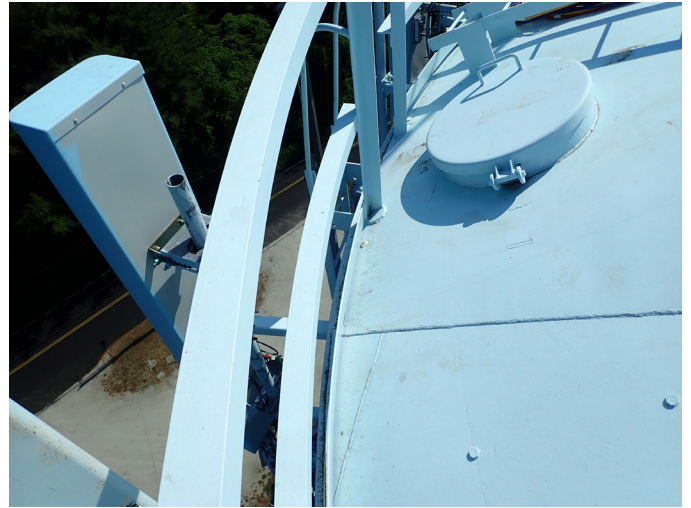
26 Pedestals Around The Vent Having Surface Corrosion
