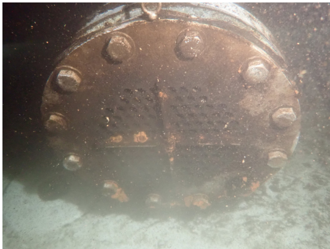
45 Unobstructed Effluent Grate And Check Valve
