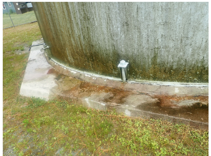
10 Exposed Foundation Having Tight Cracks And Anchor Bolt Assembly Having Good Adhesion Value Of The Protective Coating
