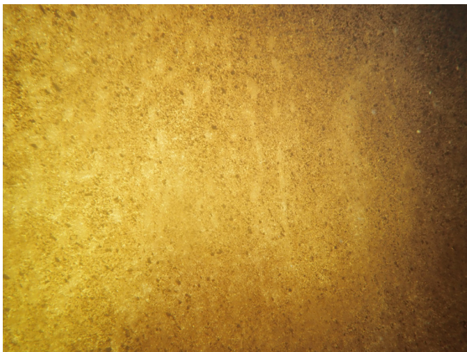
59 Interior Walls Having Good Adhesion Value Of The Protective Coating And A Mild To Moderate Stain/ Biofilm
