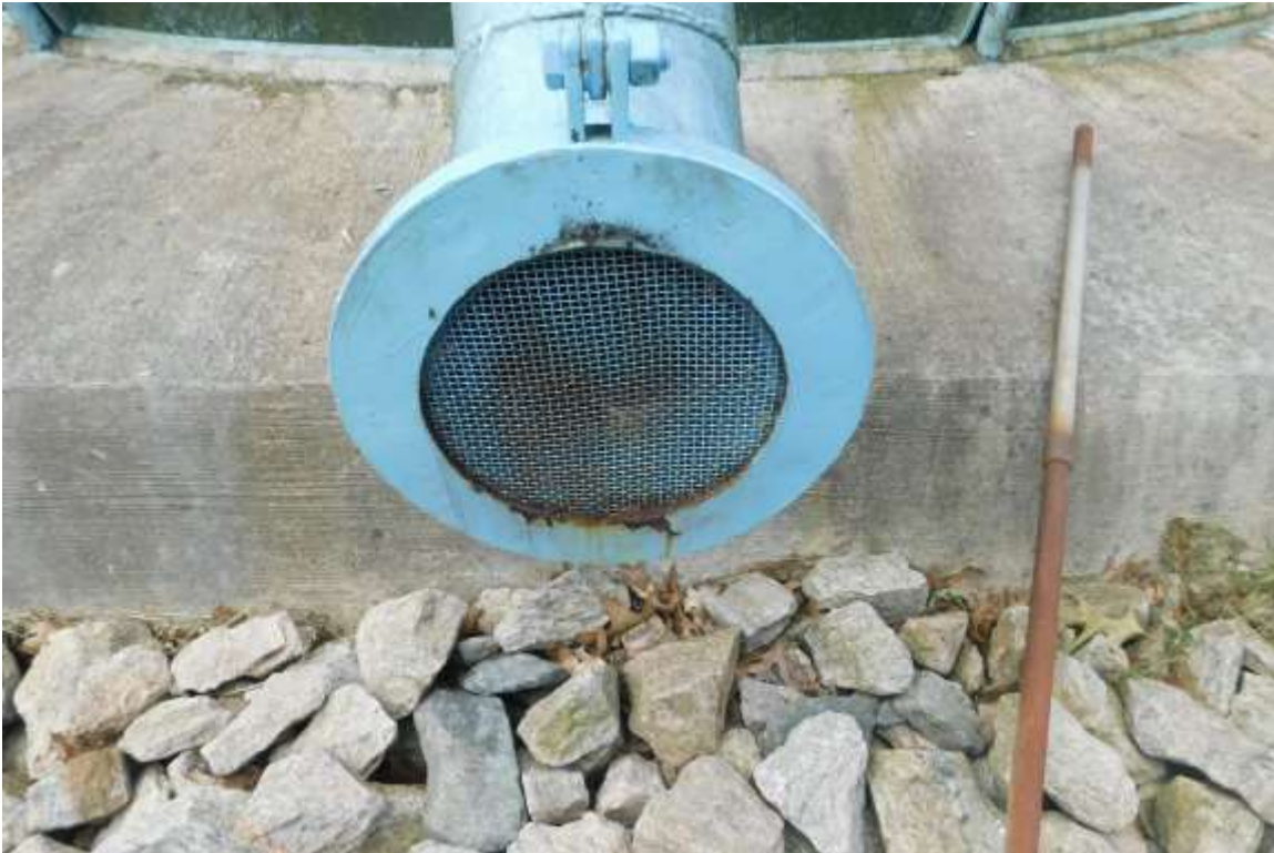
Photo shows the 10" overflow pipe system, which appears to be in good condition.
