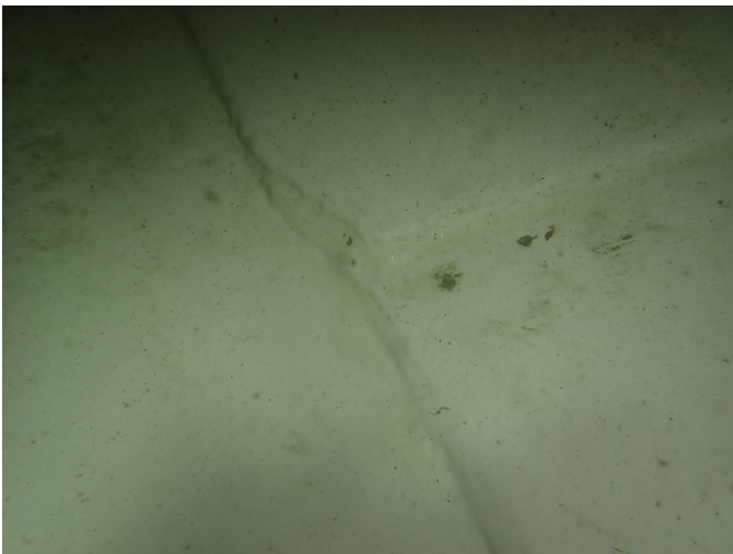
41 Floor Having Good Adhesion Value Of The Protective Coating And A Mild Stain/Biofilm
