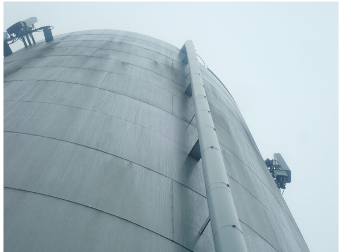
16 Overflow Pipe Having Good Adhesion Value Of The Protective Coating
